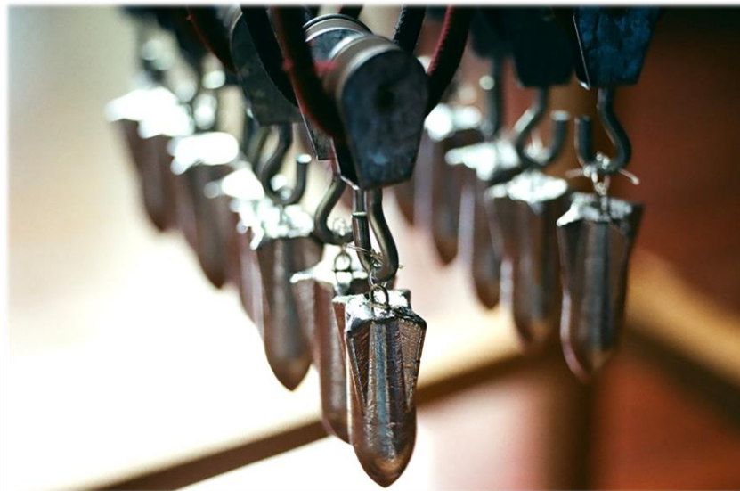
Figure 9: Cord-weights and pulleys
