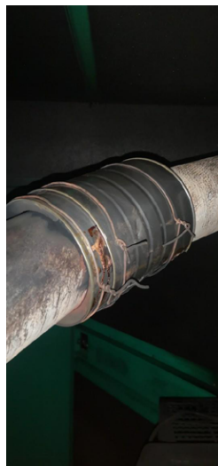
Figure 6 | Provisional patch that has become definitive for the wood-burning heater at the school. Fondecyt MaReCe, November 2021.
