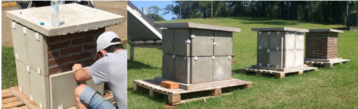
Figure 5 | Installation Facade Plates, and Finished Prototypes.
