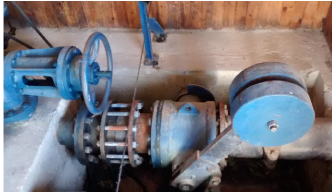
Figure 5 | Abandoned mini-hydro power plant in Puerto Edén. Fondecyt MaReCe archives, November 2021.
