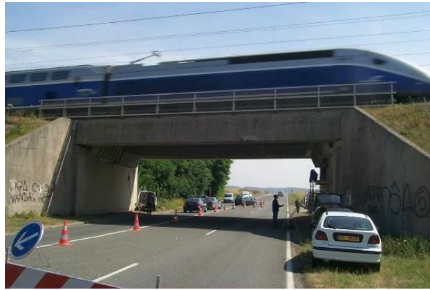
Figure 2 – Side view of the viaduct.
