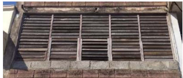
General Gómez No. 3 (1956), vanos de 4.40m x 1.70m
