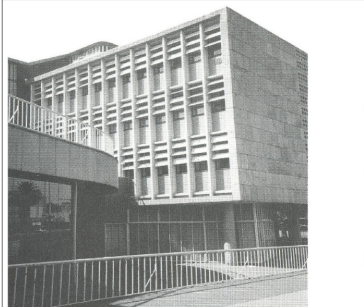
Above: Stauch's synthesis of 'Brazilian design' for the Meat Board Building (1950), Pretoria – long, modular office block raised off the lower ground slope with cylindrical pilotis , brise soleil , curvilinear roof garden, deep blue mosaic cladding of spandrels (Gerneke in Fisher et al , 1998:224).
