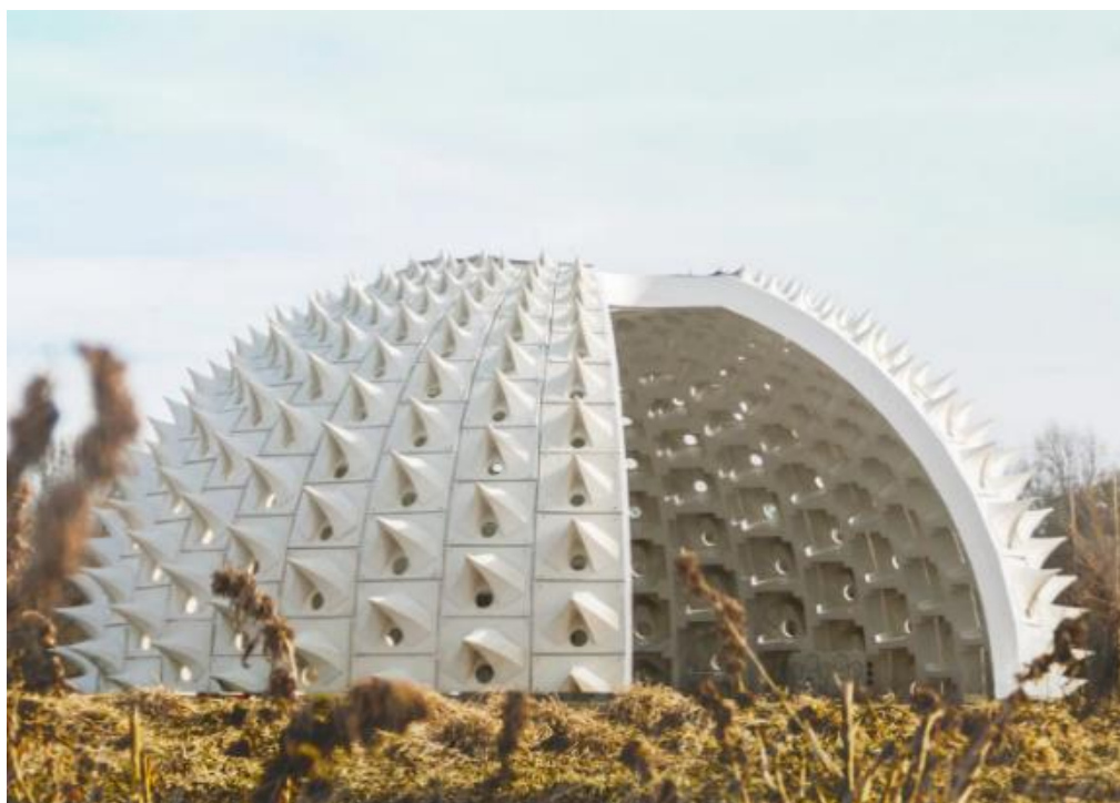
Figura 4: Pavilhão “Pollinators Pavillion”.
