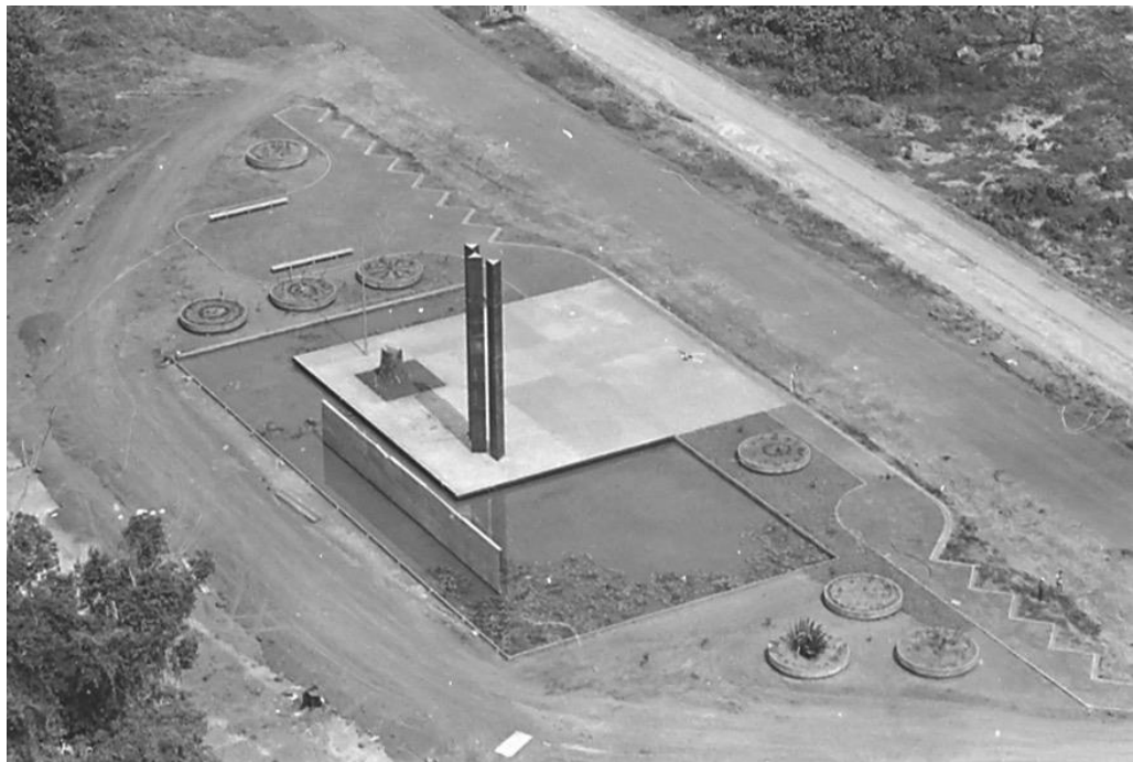
Figure 1: Monument to the Transamazonian Highway, Altamira, 1970.
