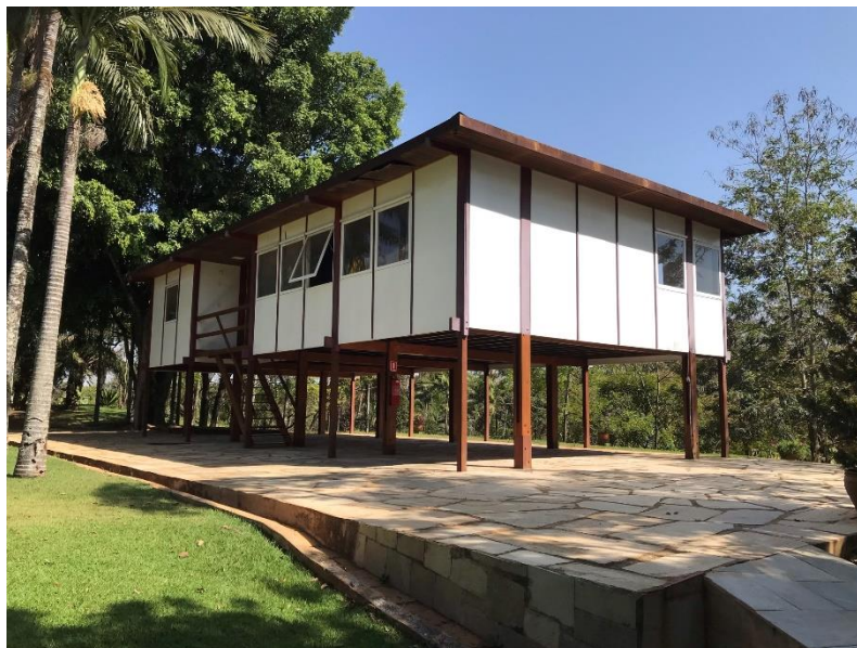
Figure 17: The pioneering headquarters of the Goiás Country Club, currently used as a memorial space for the club.
