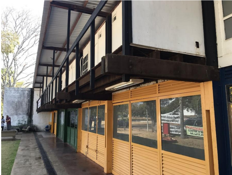
Figure 13: OCA II, housing the University of Brasília's Security Department.
