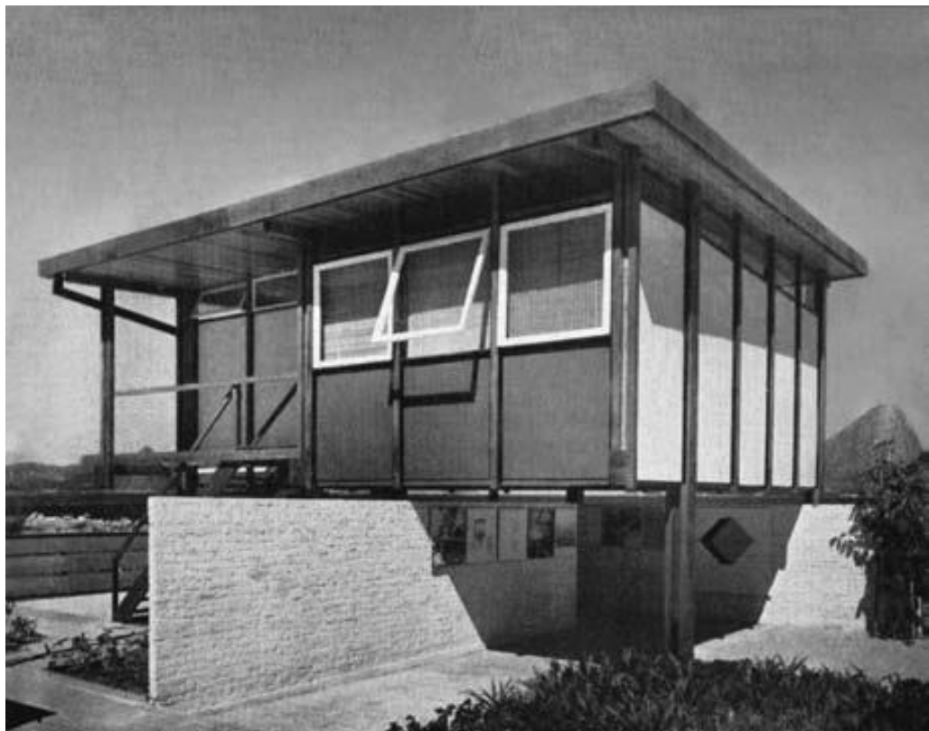
Figure 1: Prototype of the housing module in Sistema SR2 executed on a 1:1 scale in the gardens of MAM Rio, in 1960, in the exhibition Casa Individual Pré-Fabricada .
