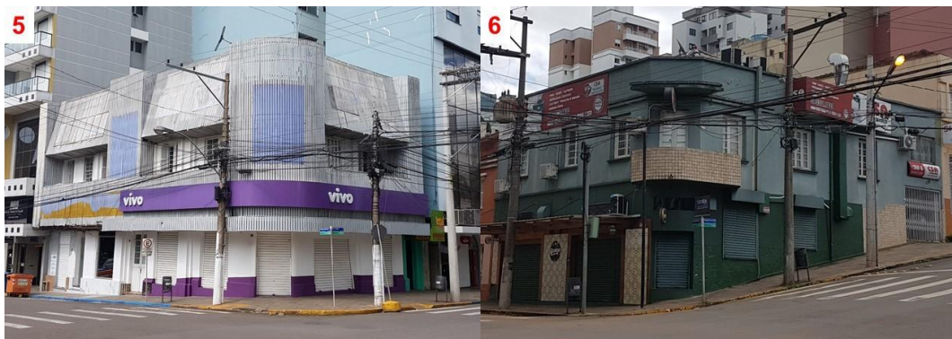
Figure 9: Buildings Nº 5 and Nº 6 presenting significant changes due to advertising activities.
