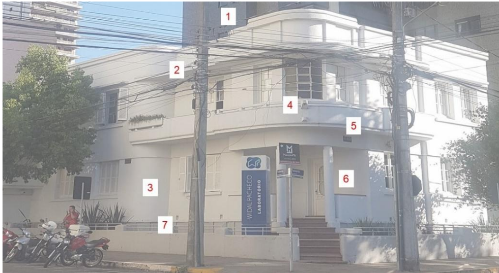
Figure 3: An Art Deco building in Passo Fundo with features demonstrating streamline moderne references, which are: cornice, marquee, curved wall and balcony (numbers 1, 2, 3 and 5); columns and flagpole support (numbers 6 and 4); and railings with circular iron profiles (number 7). It may be noted that, in this case, all the circular elements of the house, added to the columns and the mast, help to demarcate the corner.
