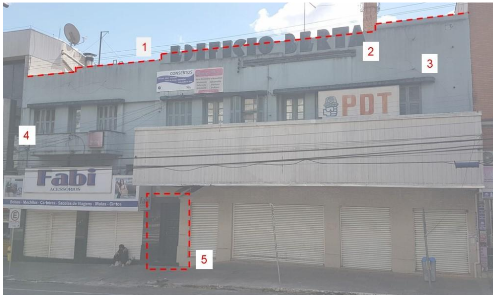
Figure 2: An Art Deco building in Passo Fundo with features demonstrating zigzag moderne references, which are: 1 - straight and staggered cornices; 2 - linear friezes; 3 - straight marquees; 4 - straight, simple volumes along the balconies; and 5 - a centralized main access, even if slightly shifted to the left.
