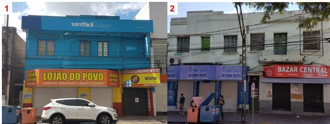
Figure 7: Buildings Nº 1 and Nº 2 presenting significant changes due to advertising activities.
