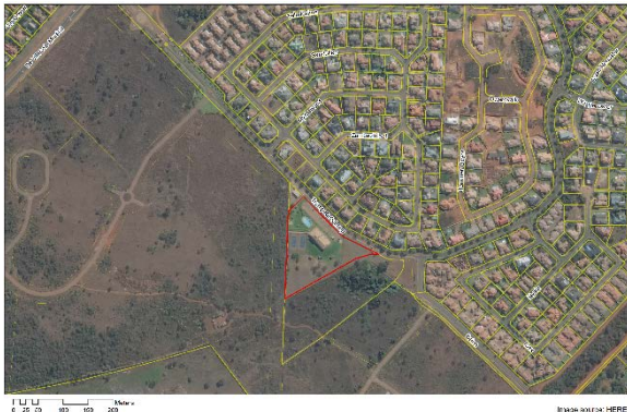
Figure 16: Form of common open space in The Wilds (Source: Map produced by Darren Nel)
