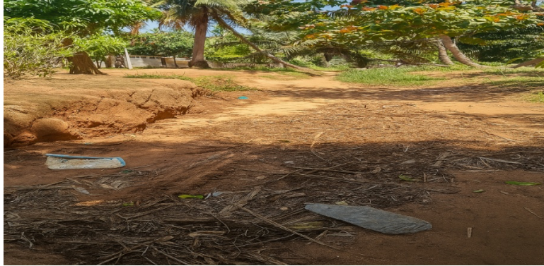
Figure 6. Formation of a gully on the access road of the 21 de Abril neighborhood. Source: Author's elaboration (2023)
