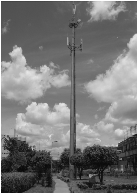
Picture 1 – Compact metal tower
