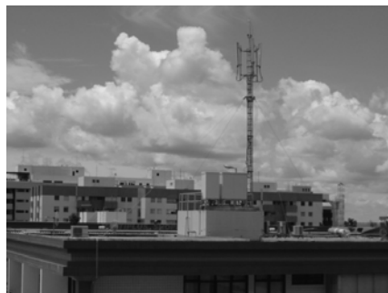
Picture 3 – Roof top metal lattice
