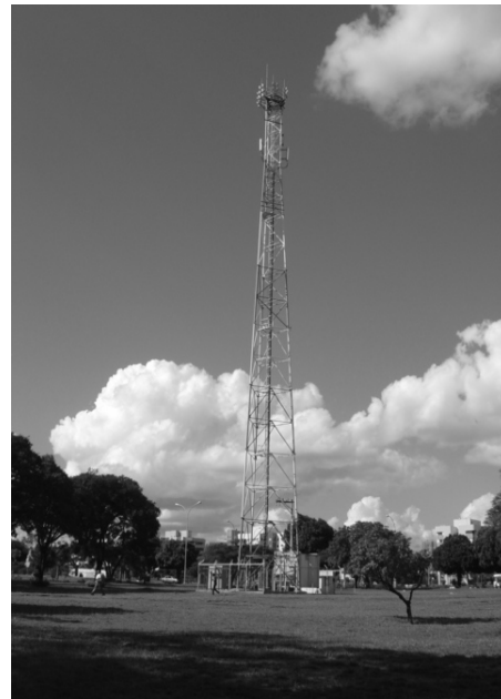
Picture 2 – Metal lattice tower
