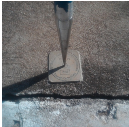
Figure 1 . Spiked plate on stable surface.
